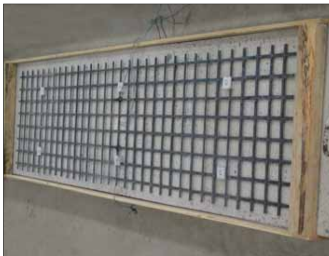
Fig 3.5 Strengthening of CFRP Grid
