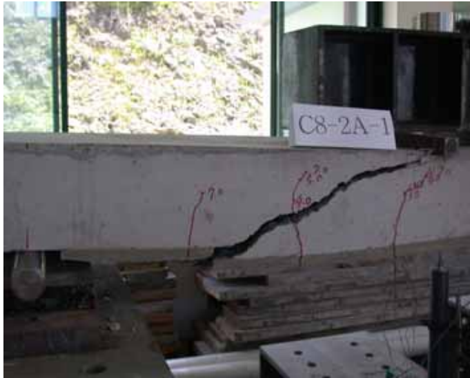
Fig 4.7 Diagonal shear failure
