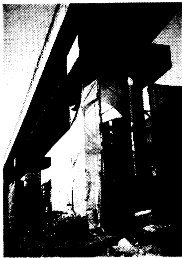
Fig. 2.7 Strengthening examples using FRP sheets(2)
