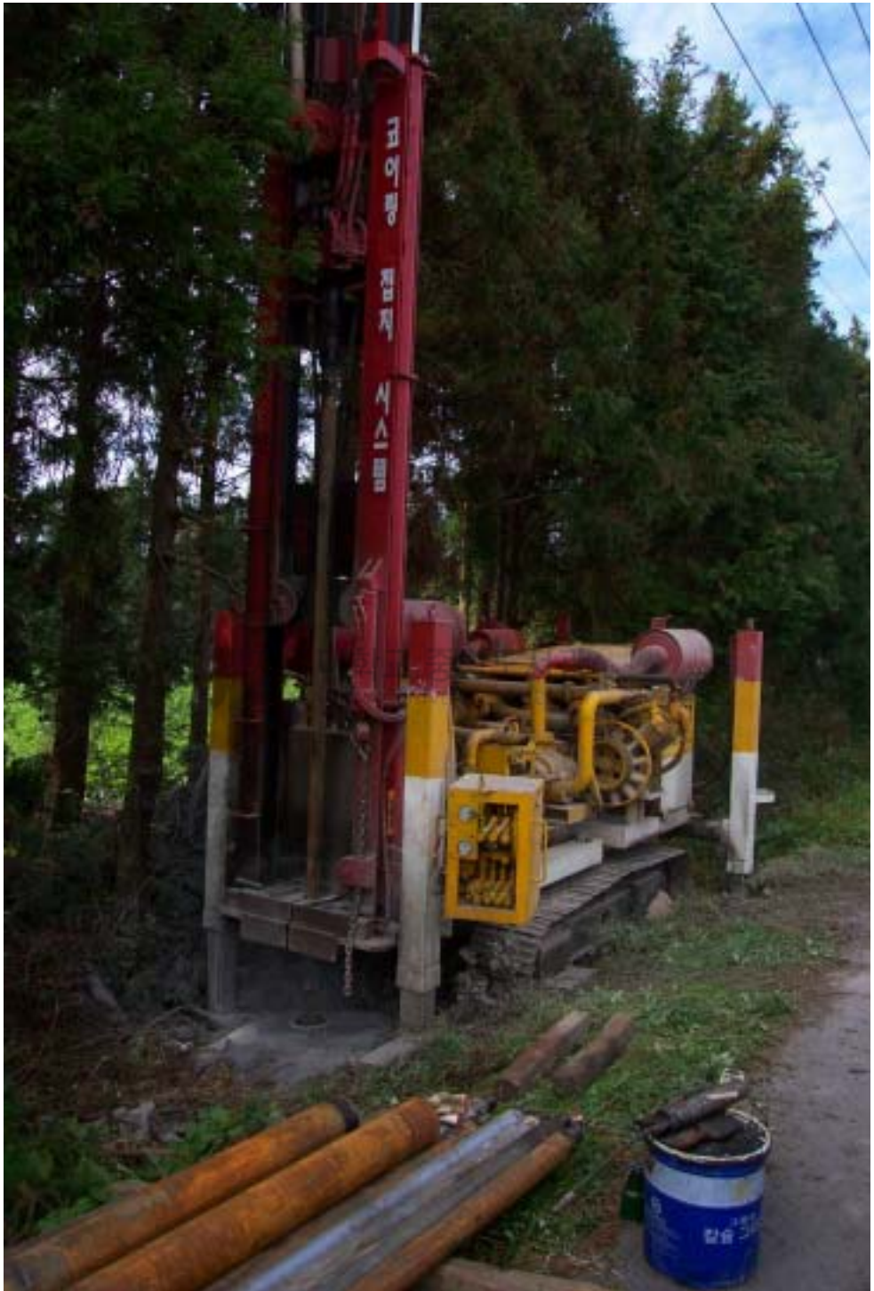
Fig. 10 Photography of coring grounding construction
