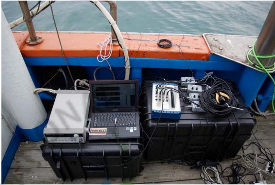
Fig. 38 SBL system Field test installation
