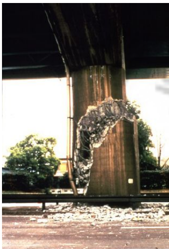
Fig. 1.1 Shear failure of pier by earthquake
