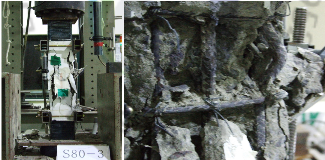
(a) Final failure and crack
