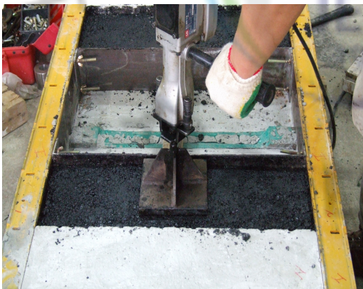
(g) Placing of asphalt concrete
