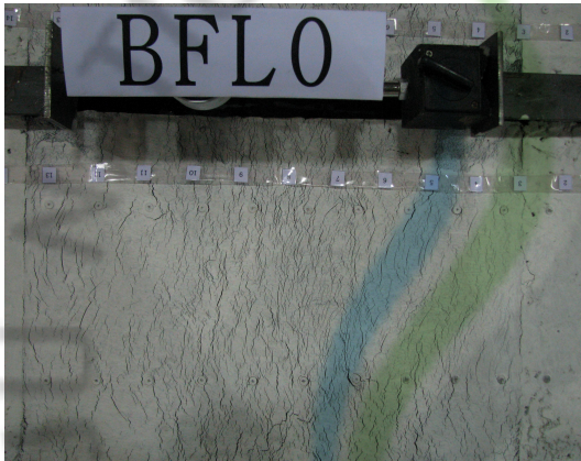
(b) Deformation patterns at surface
