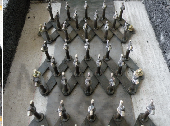
(b) Installation of bottom system
