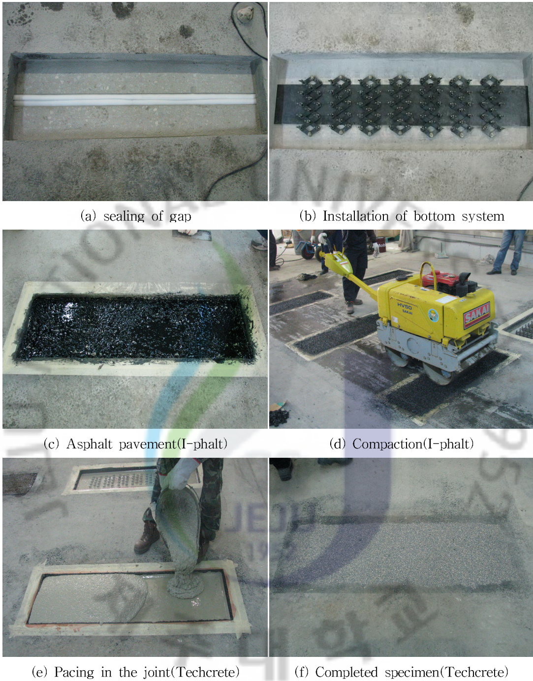
Fig. 4.20 Manufacture process of joint
