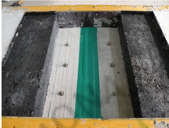
(a) sealing of gap
