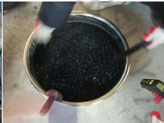
(d) Mixing of aggregate and asphalt
