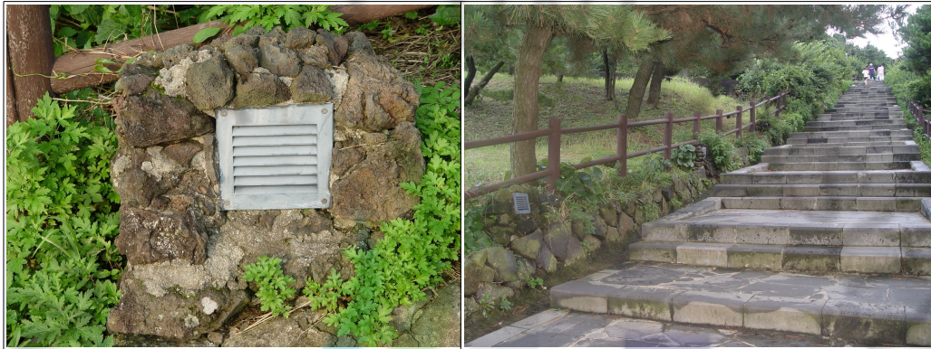
Fig. 4 External appearance of installed luminaire at wide stair section
