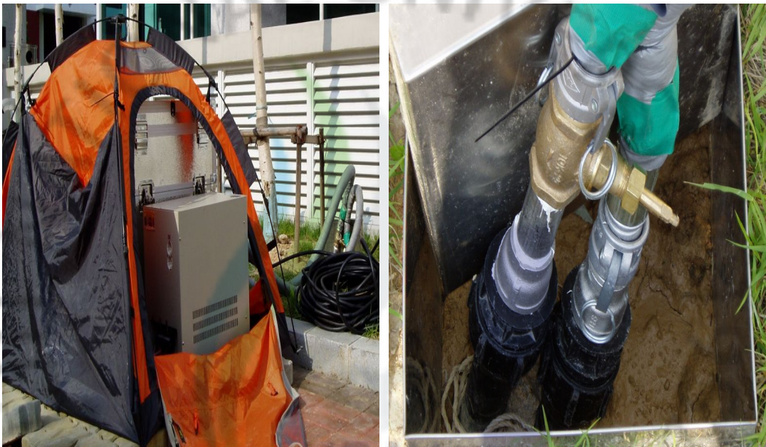
Fig. 12 The picture cTRT and geothermal heat exchange loop at KIER
