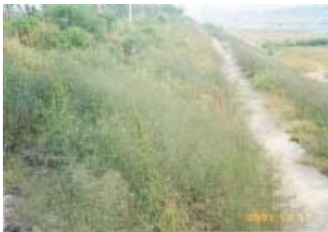
Fig. 5-16. High-flow revetment in Anyang Stream
