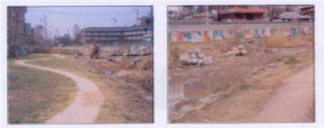
Fig. 5-25. Esplanade on the waterside Fig. 5-26. Natural stone revetment
