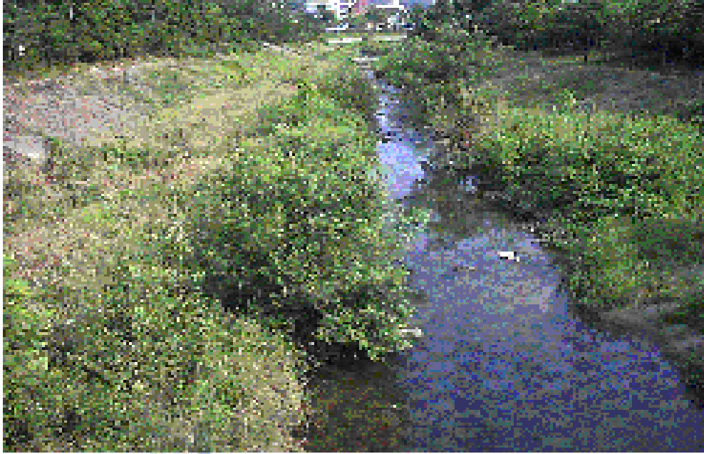
Fig. 5-3. Low waterway and high level berm(April, 2000)
