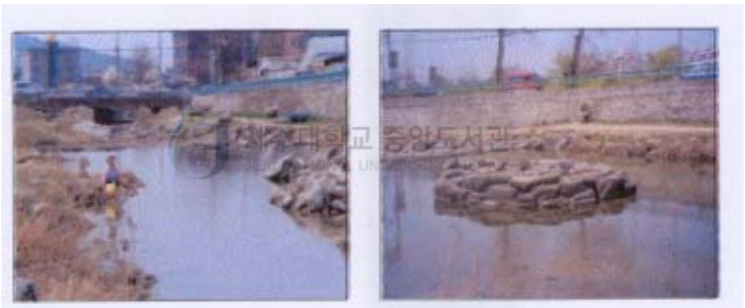
Fig. 5-27. Feature of decoration with natural stone revetment
