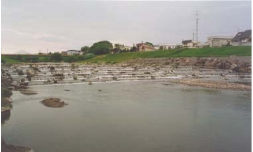
Fig. 6-4. Fish stream of Chitose made stone the whole surface fish way
