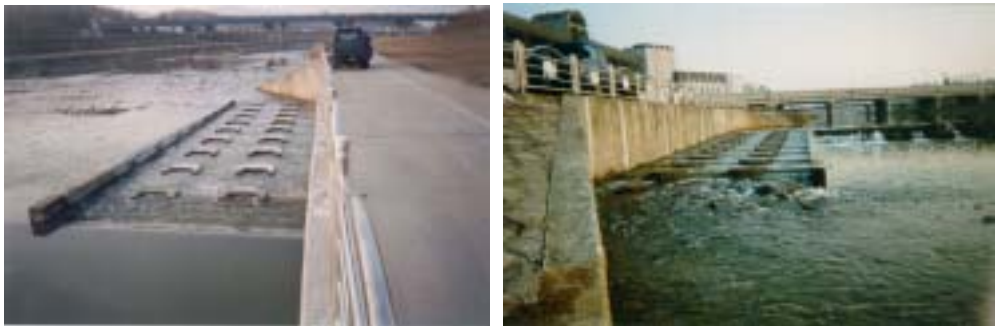
Fig. 6-9. Fish way facility of downstream of Tan Stream (after water flow)
