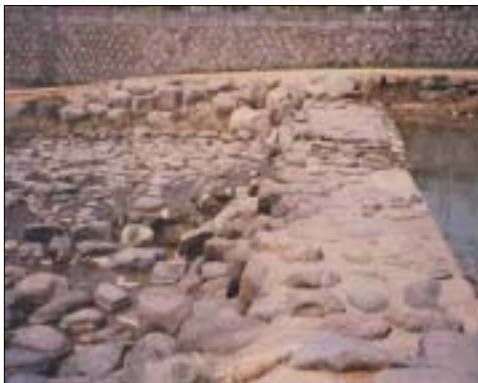
Fig. 5-23. Falling works with use of natural stones and concrete
