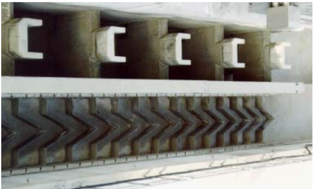
Fig. 6-3. Muromathbara Iceharbor type & pass type Denill type fish way
