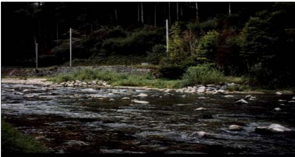
Fig. 4-3. Sihl River protected with groyne of railway side
