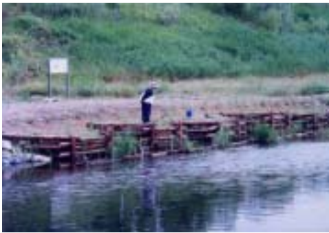
Fig. 5-18. Plantation zone of filtration
