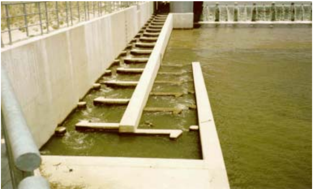
Fig. 6-5. vertical slot type fish way of Muromathbara
