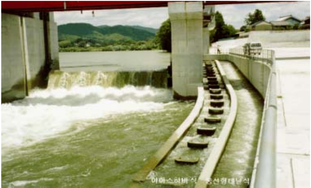
Fig. 6-6. Muromathbara iceharbor type fish way & pass type Denill type fish way
