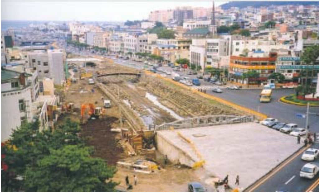
Fig. 5-32. Feature of restoration work of Sanji Stream in Jeju City
