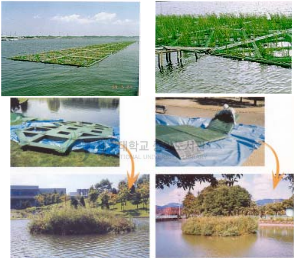
Fig. 6-11. Installation of water plant cultivation island in Japan
