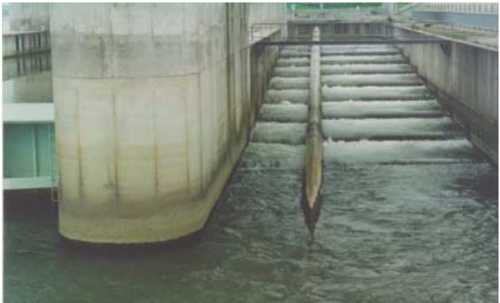
Fig. 6-7. Stepped type fish way of Ojima
