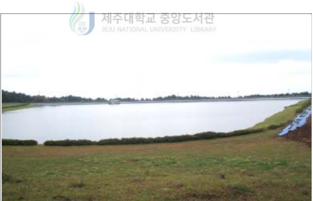
Fig. 5-3. Overall view of Eoseungsaeng dam
