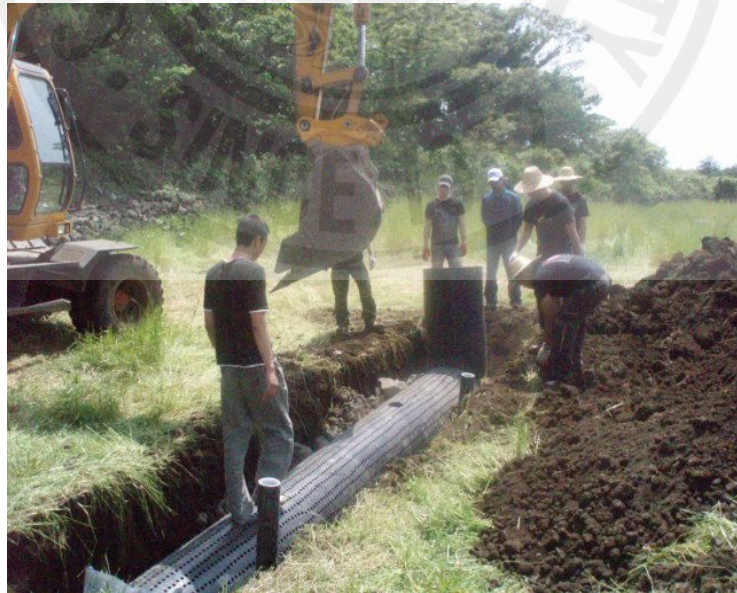
Fig. 4.6 Installation of an infiltration trench
