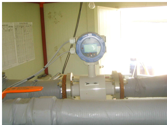
Fig. 3-6 The installation of the flow meter
