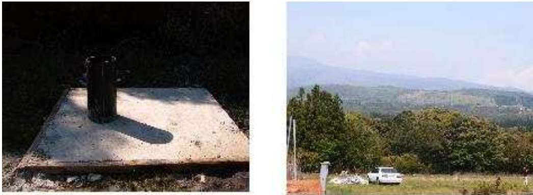
Fig. 2-3 The photo of the boring point
