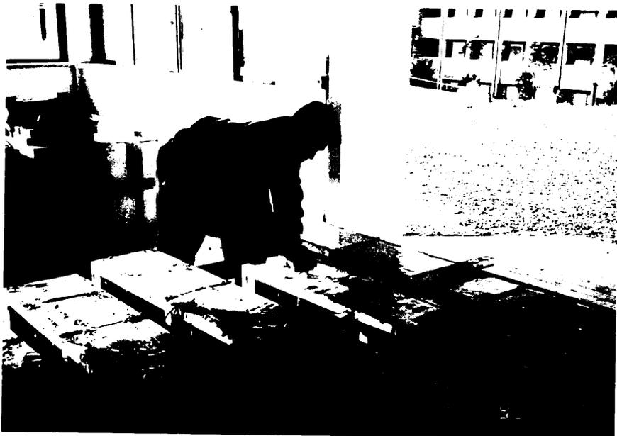
Photo 4 Finishing of concrete
