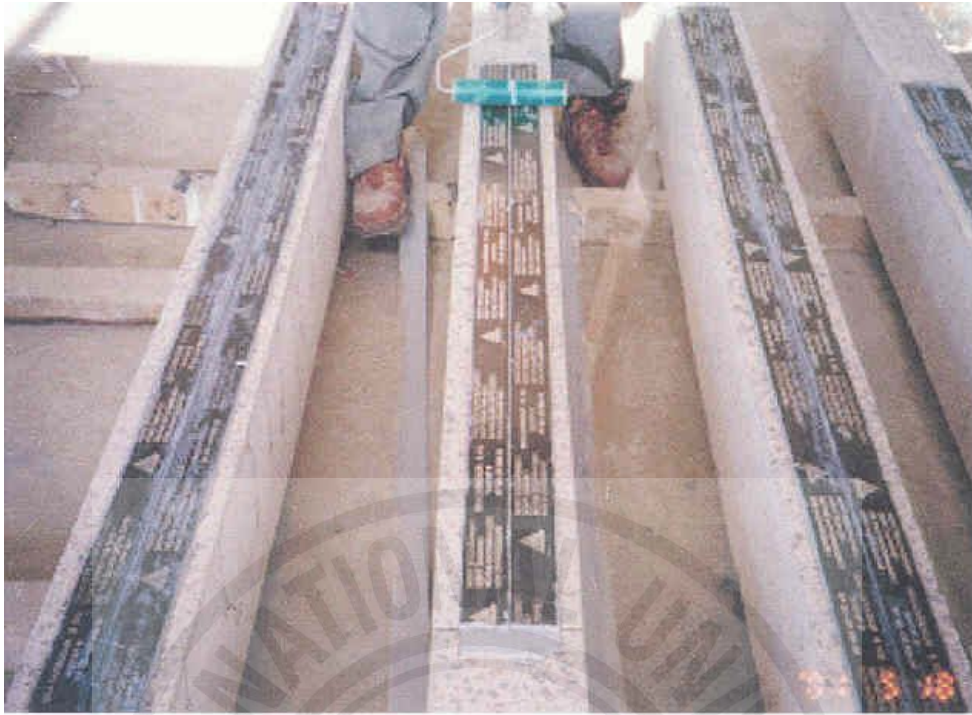
Fig. 3.12 Roller pressing on CFRP plates
