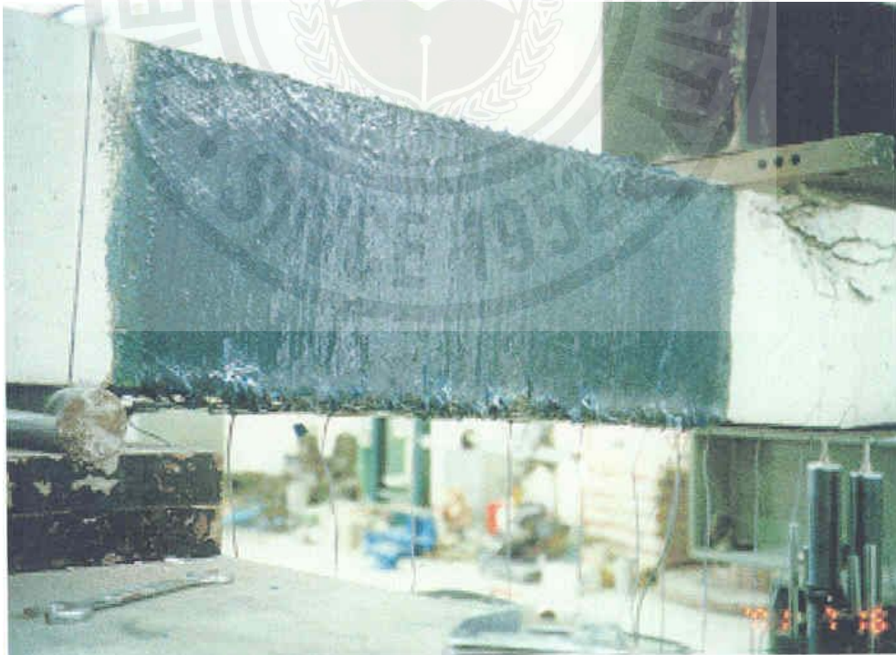
Fig. 4.23 Delamination shear failure of beam FPL3
