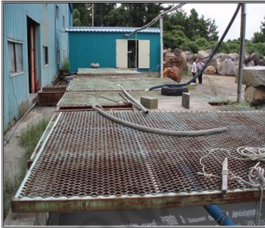
⑤ 3rd Settling
