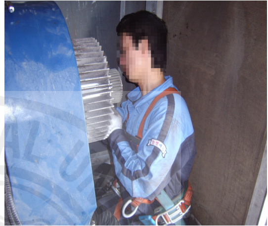
Fig. 32 The work changing VRCC control unit
