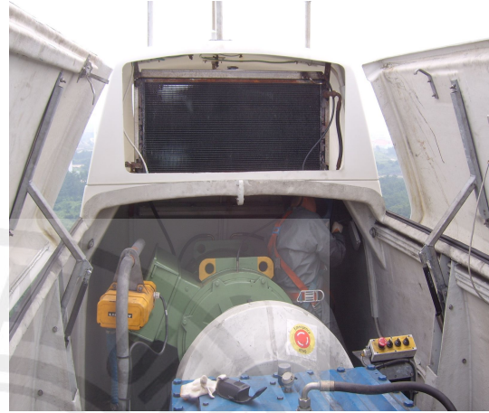
Fig. 38 The work changing anemometer on the nacelle
