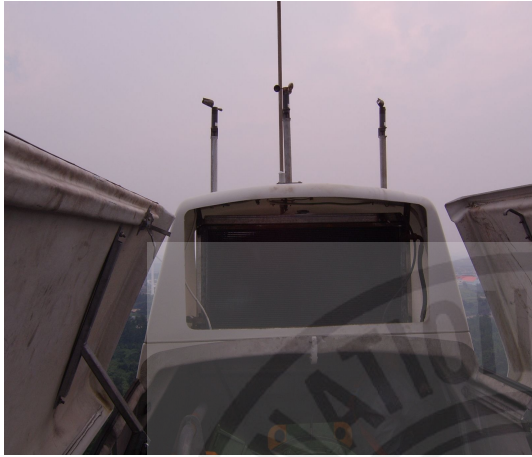
Fig. 37 The picture of anemometer on the nacelle
