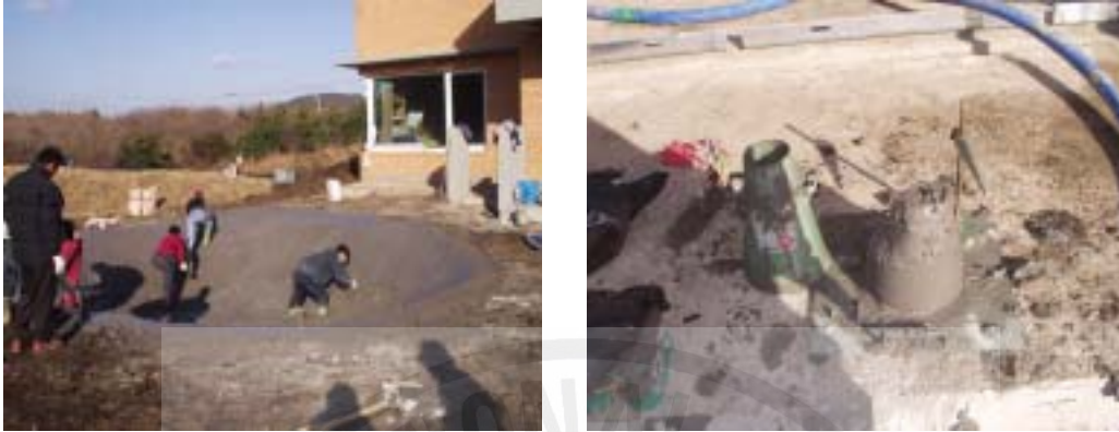
Fig. 6.12 The Pond Construction Process using Powered Basalt Sludge (Finishing, Slump Testing)
