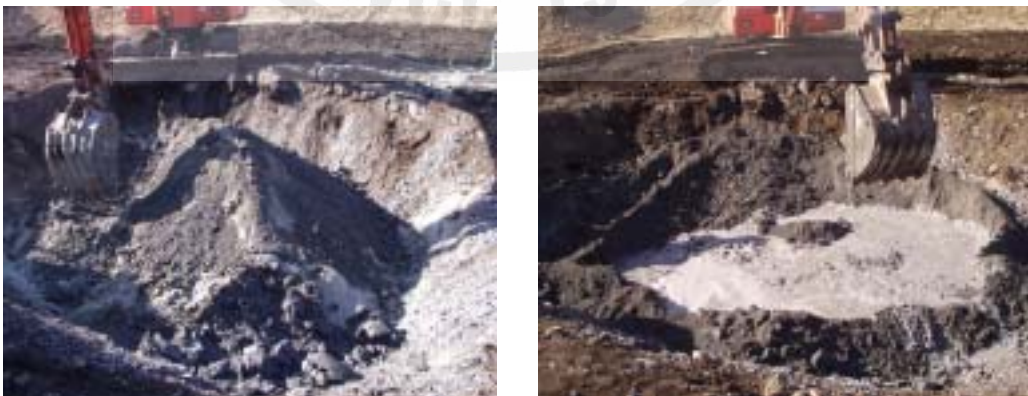
Fig. 6.11 The Pond Construction Process using Powered Basalt Sludge (Mixing-2, Mixing-3)
