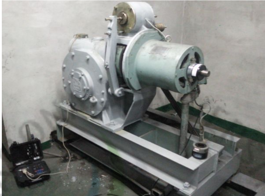
Fig. 5.18 Measurement of vibration
