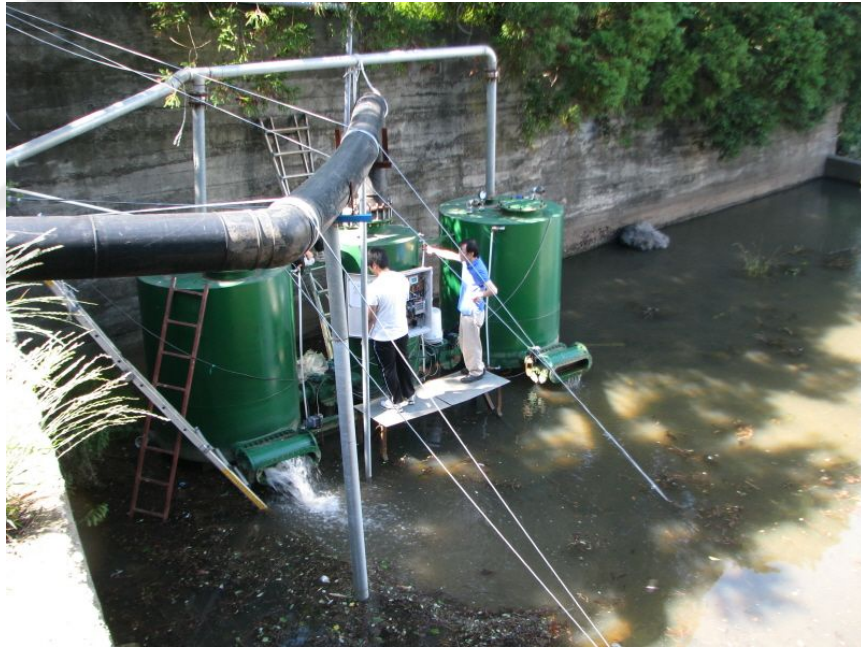
Fig. II-26 Condition of in-pouring at left chamber
