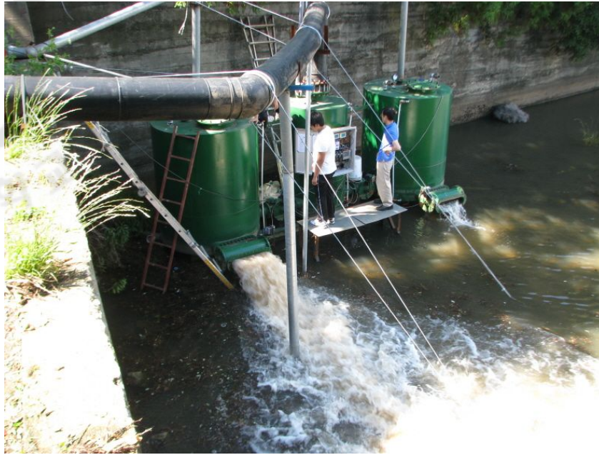
Fig. II -27 Water discharging situation at left chamber
