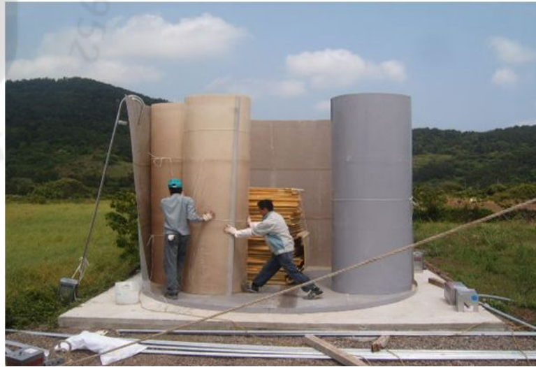
Fig. 4. Heat storage tank under construction.
