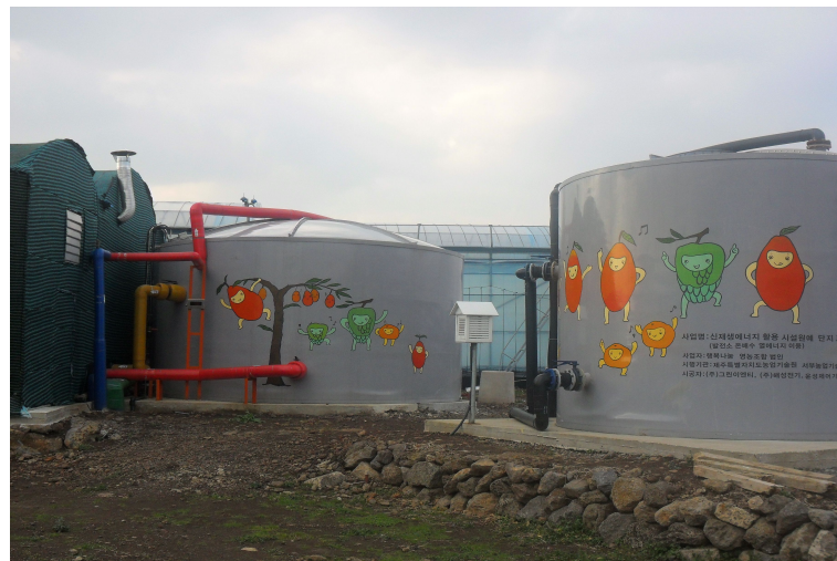
Fig. 5. Completed heat storage tank.
