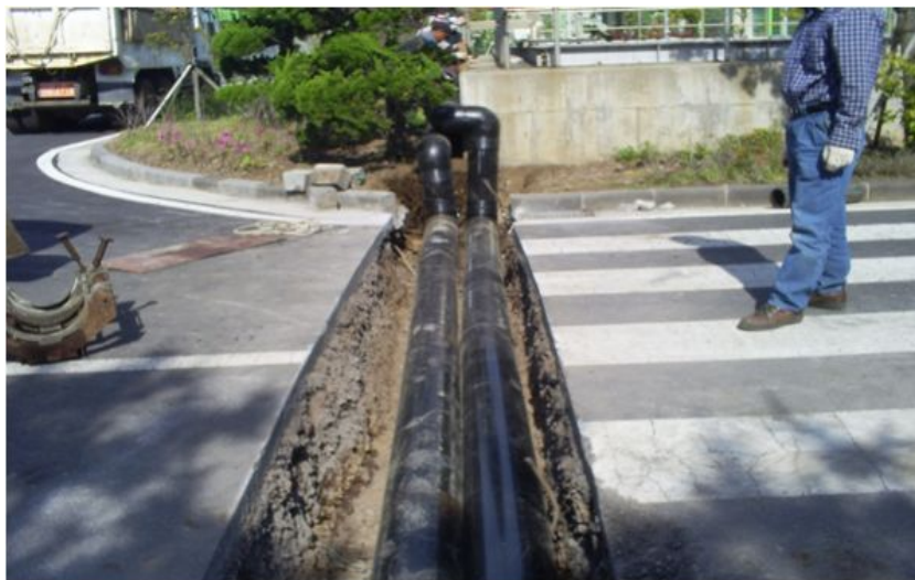
Fig. 8. Installation of the pipelines to convey saltwater.
