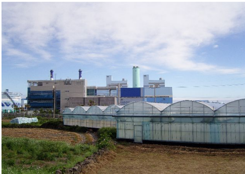
Fig. 1. The view of Korea Southern Power Plant and the laboratory for the experiment on the use of hot waste water.
