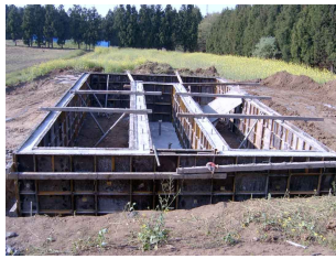
Construction of experimental field
