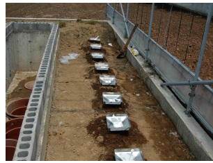
Installing of lysimeter
