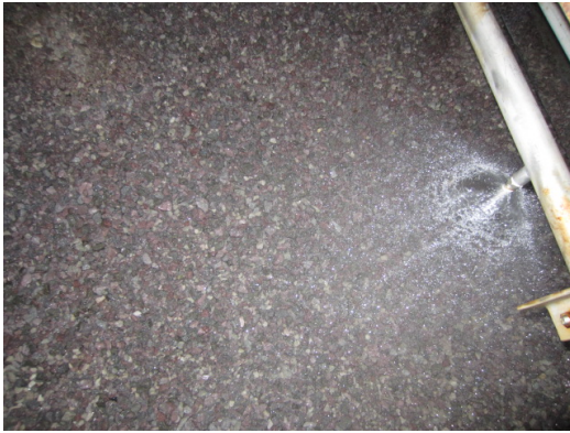
(a) Good example (spray over packing material)
