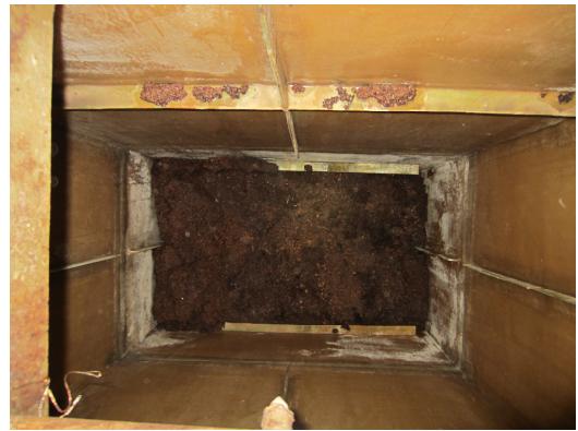
(d) Poor example (reduced height of packing material)
