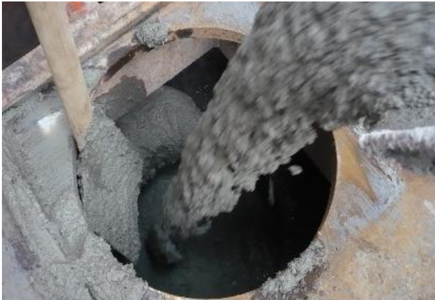
Fig. A2 The grouting
