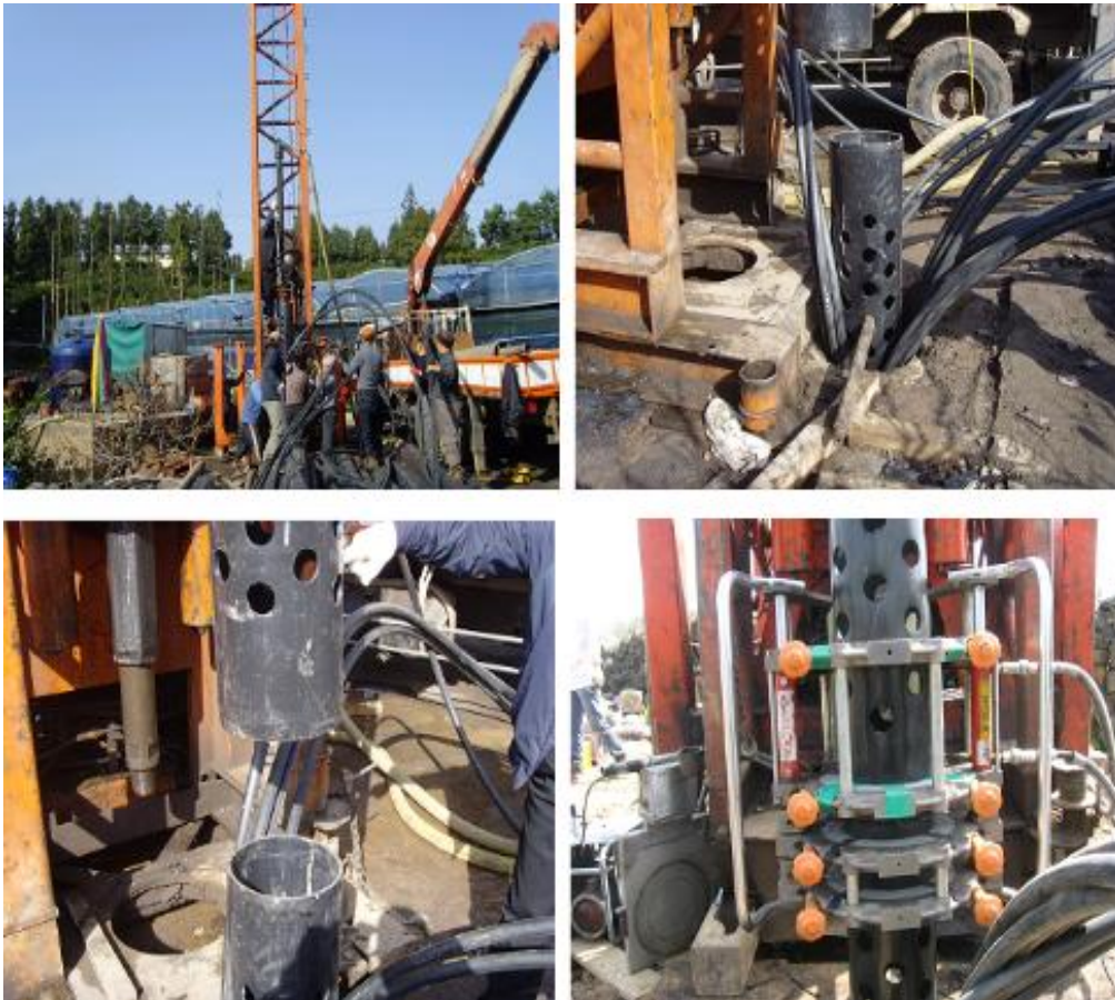
Fig. 7 The boring and underground heat exchanger installation
