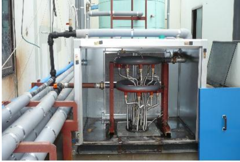
Fig. A3 The geothermal heat exchanger
