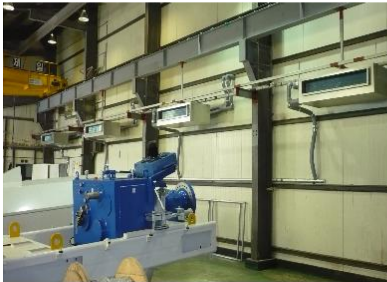
(b) Industrial building
