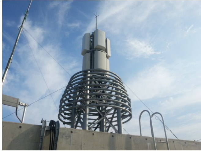
<Figure 13. TV broadcasting Antenna>
