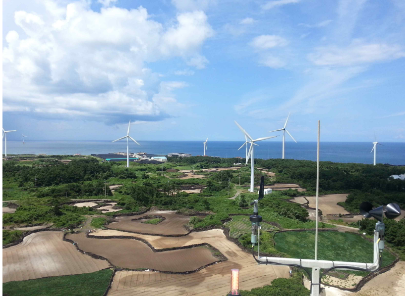
Fig. 35 Hangwon wind farm.
