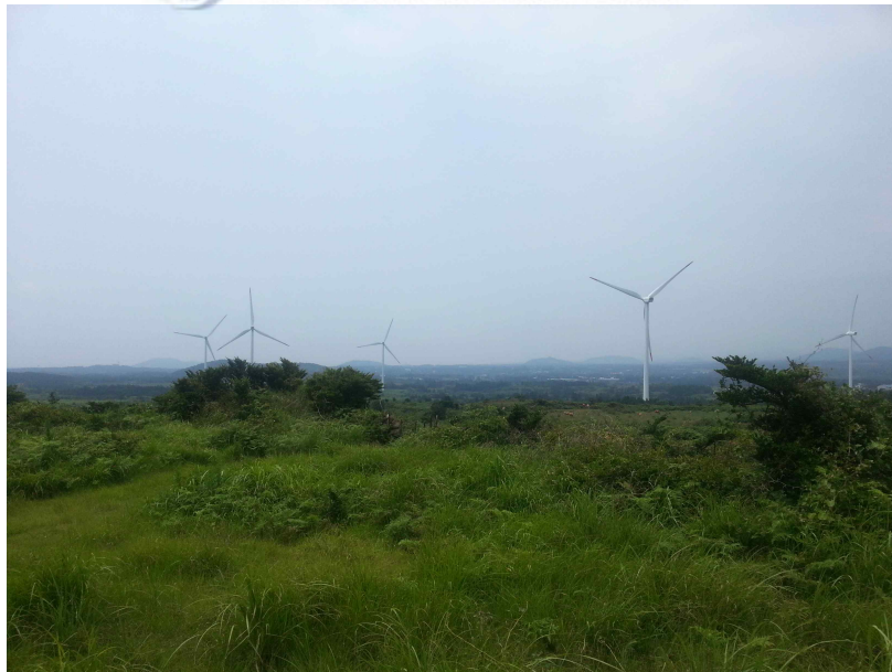
Fig. 36 Samdal wind farm.
