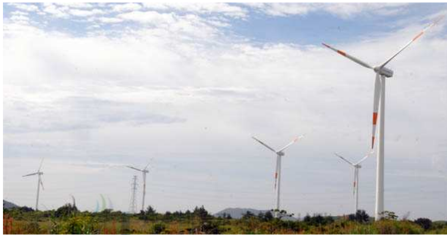
Fig. 29 View of WTG under test in Seongsan wind farm
