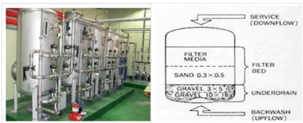
Fig. 17. The mimetic diagram of multiple media filters
