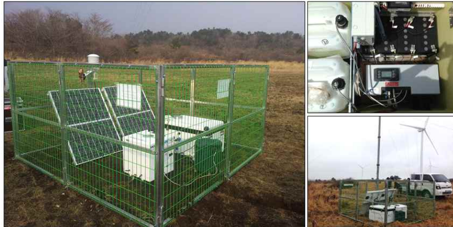
Fig. 2-5 Ground-based LiDAR installation at a site
