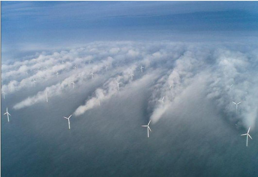
Fig. 1.3 Wake effects in wind farm(Horns Rev 1)[2]
