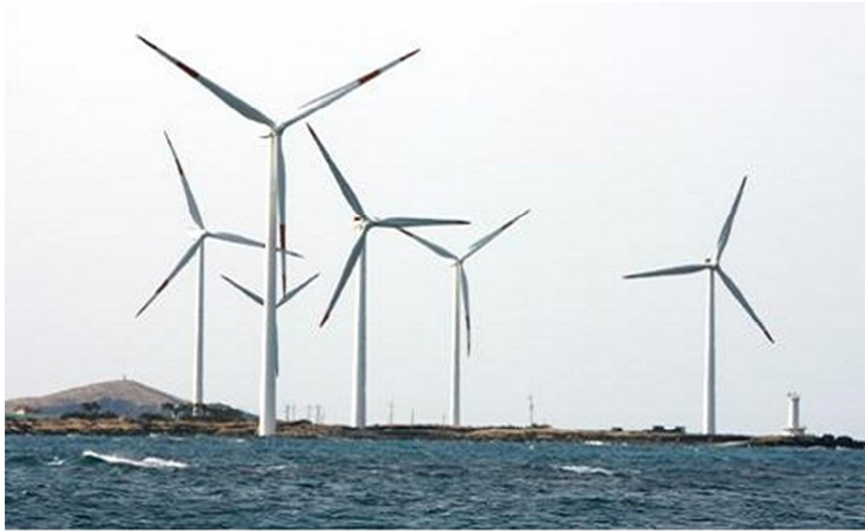
Figure 5-2 View of wind turbines under test in Hankyeong wind farm
