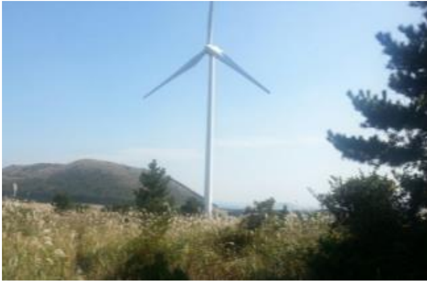
Figure 3-2 View of the wind turbine under test in Gasiri wind farm
