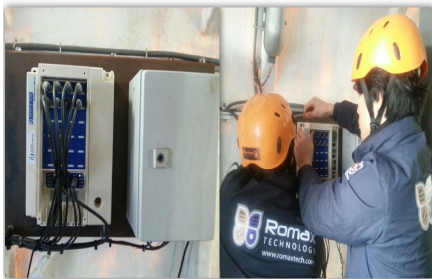
Figure 1-1 Installation of condition monitoring system
