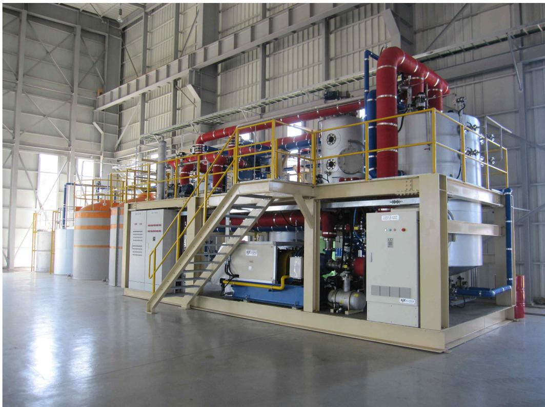
Fig. 4-11 MVR desalination plant
