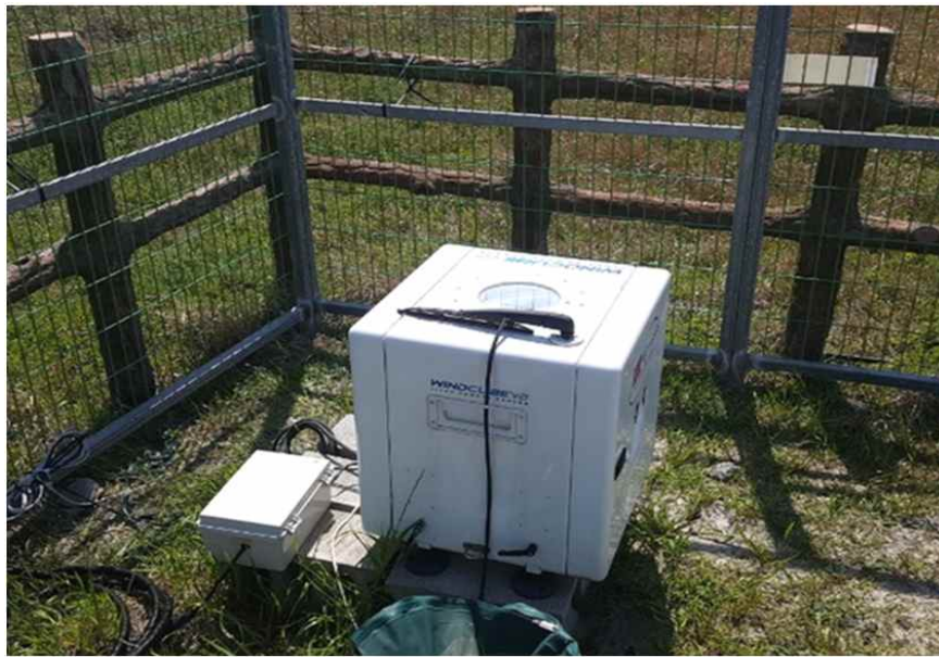
Fig. III-11 Ground LiDAR installed at the Haengwon wind farm
