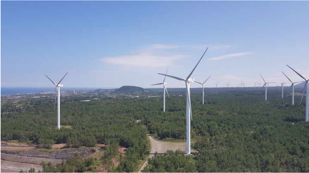
<View seen at the nacelle of Dongbok wind turbine no. 1 (photograph by D. H. Shin)>
