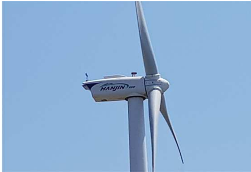
Fig. III-4 View of test wind turbine at the Haengwon wind farm
