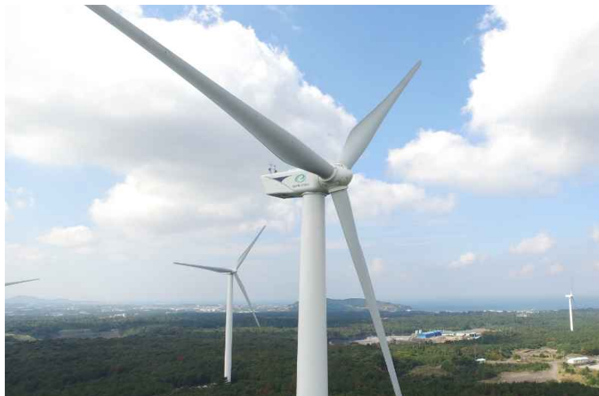
Fig. IV-8 View of the test wind turbines at the Dongbok wind farm
