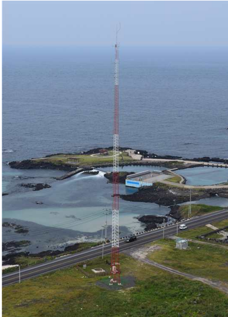
Fig. III-14 Met mast installed at the Haengwon wind farm
