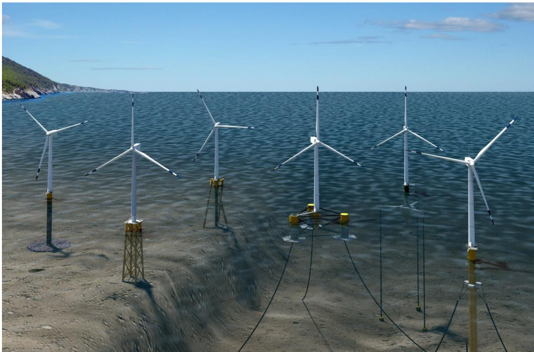
Figure 1.4 Offshore wind turbines: bottom-fixed type (three from left) and floating type (three from right) [4]
