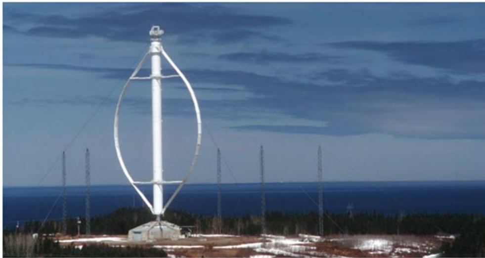
Figure 1.10 4MW Darrieus VAWT, Éole, on the north shore of Quebec's Gaspé peninsula [12]
