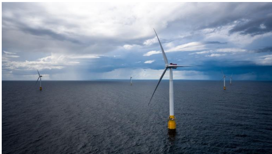
Figure 1.8 30-MW Hywind Scotland Pilot Park [10]
