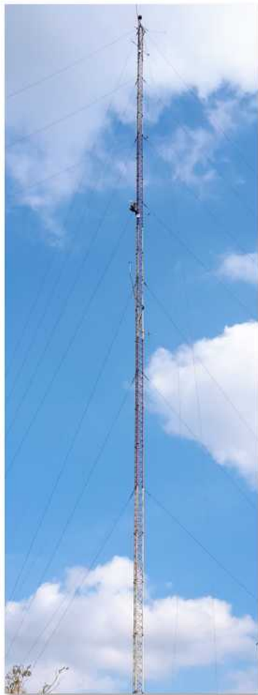
Fig. 2.2 A view of the 80m tubular-type meteorological mast installed at the Dongbok-Bukchon wind farm in Jeju Island
